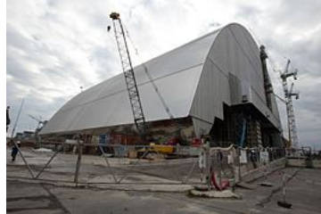
Nearing completion in October 2016
