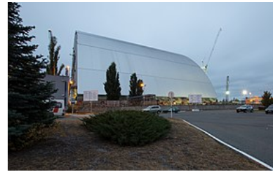
The NSC nearing completion in October 2016
