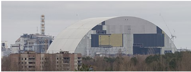
Construction in March 2016
