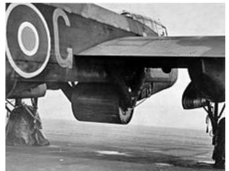
"Upkeep" bouncing bomb mounted under Gibson's Lancaster B III (Special)
