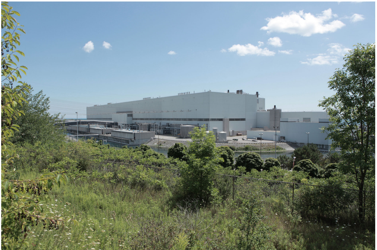
Darlington Nuclear Generating Station, 2012-08-01, photo by Milan Ilnyckyj
